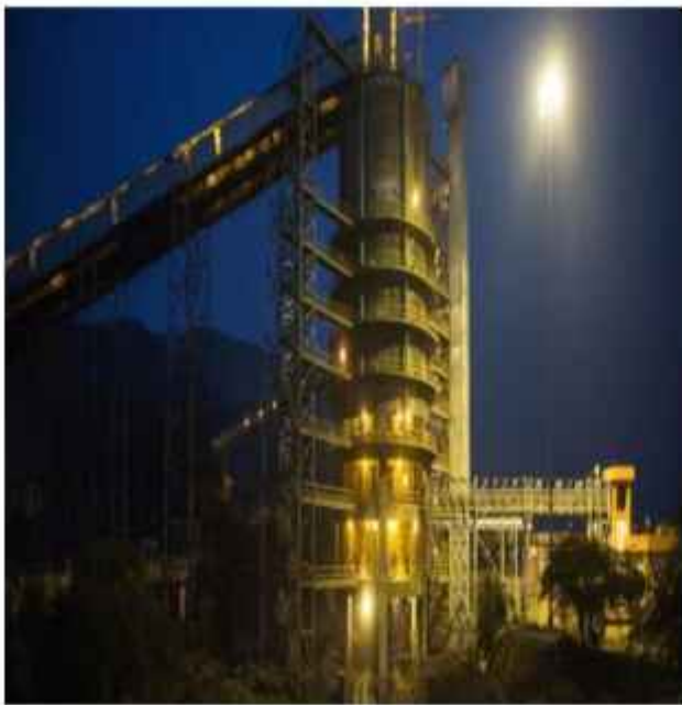
Amlohri CHP at NCL
