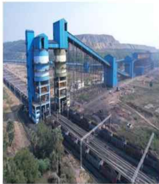
CHP (10 Mt) Built at Sattupally, Telangana
